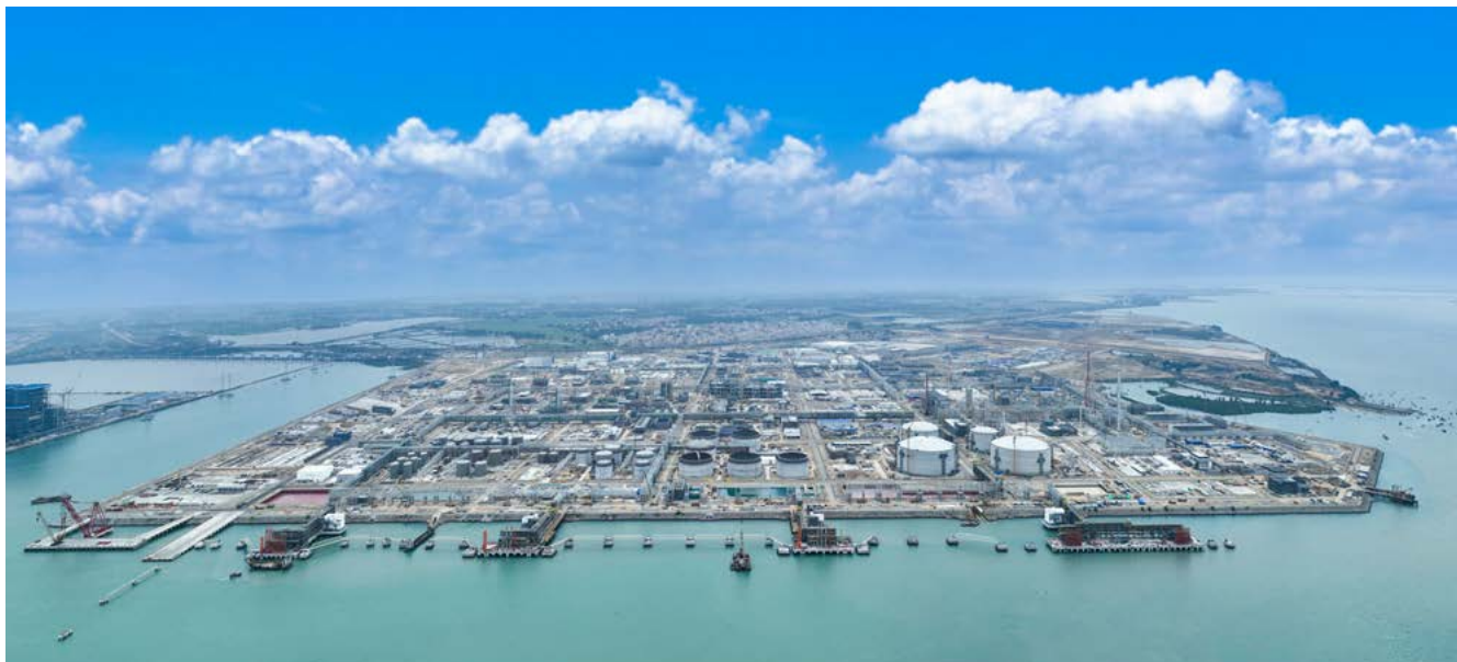
Construction in progress at BASF's Zhanjiang Verbund site (status April 2024)
