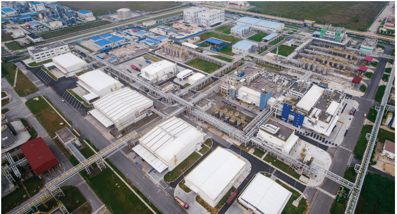
BASF Shanghai Caojing site; BASF Shanghai Coatings Minhang and Caojing sites, and BASF Coatings' resin plant in Caojing, Shanghai, realized 100% renewable energy usage across its operations in 2023.
