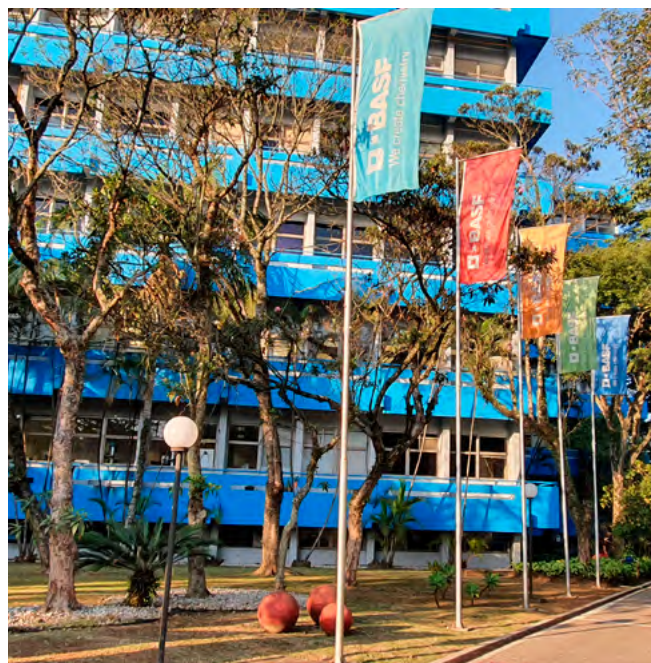
BASF's Industrial Paints and Varnishes Complex in São Bernardo do Campo (SP, Brazil)
