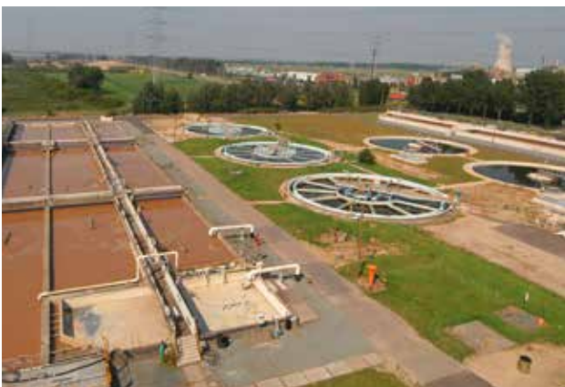
Our water treatment facility has the capacity to treat the water of a city like Antwerp.
