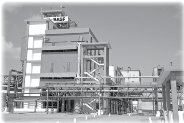
The Dispersions plant with expanded capacity is ready to cater to the growth in the user industries, such as paper, construction, paints and adhesives.
