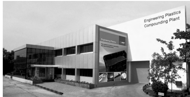
Newly opened BASF's Engineering Plastics Compounding Plant and the Computer Aided Engineering (CAE) Centre at Navi Mumbai site.
