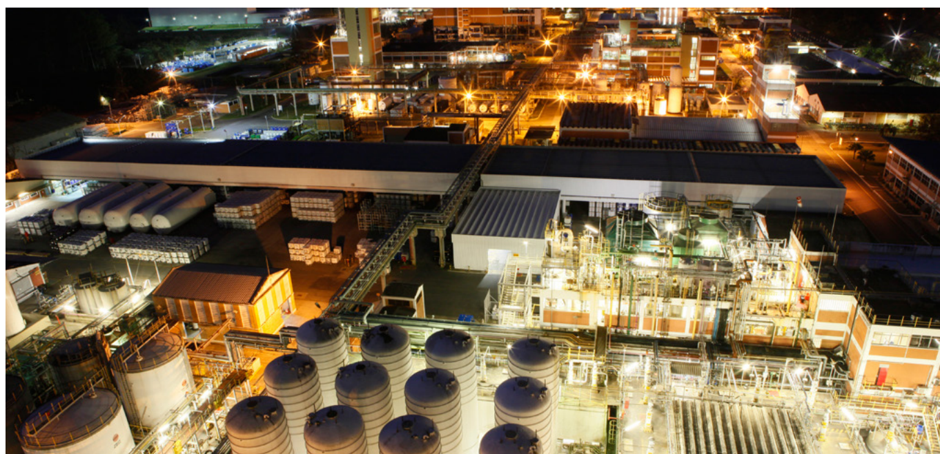
Chemical Complex in Guaratinguetá (SP, Brazil)
