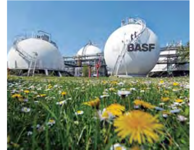
Tank storage facility at Friesenheim Island section of BASF's Verbund site in Ludwigshafen.
