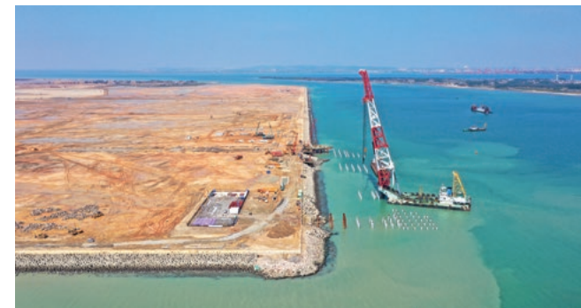
Construction in progress at BASF's new Verbund site in Zhanjiang
