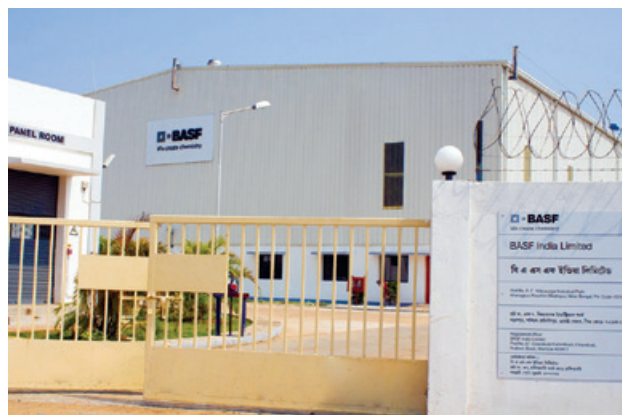
BASF's new concrete admixtures plant, located in Kharagpur, West Bengal
