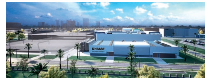
The photo shows a 3D simulation of the first plants of the Verbund site in Zhanjiang.
