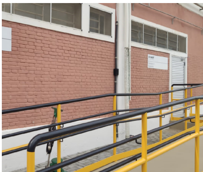
Accessibility ramp for People with Disabilities
