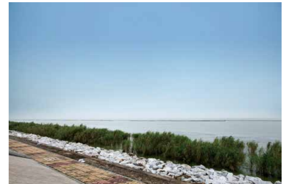
Passive House Bruck was built by Taihu Lake that suits the typical climate condition in the Yangtze River Delta region.
