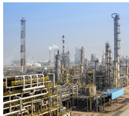
BASF and Sinopec operate the Verbund site BASF-YPC Co., Ltd., in Nanjing, China, a 50-50 joint venture.
