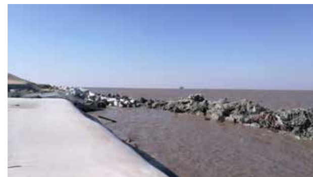
Elastocoast slope protection system is used at Hengsha Island in Shanghai.
