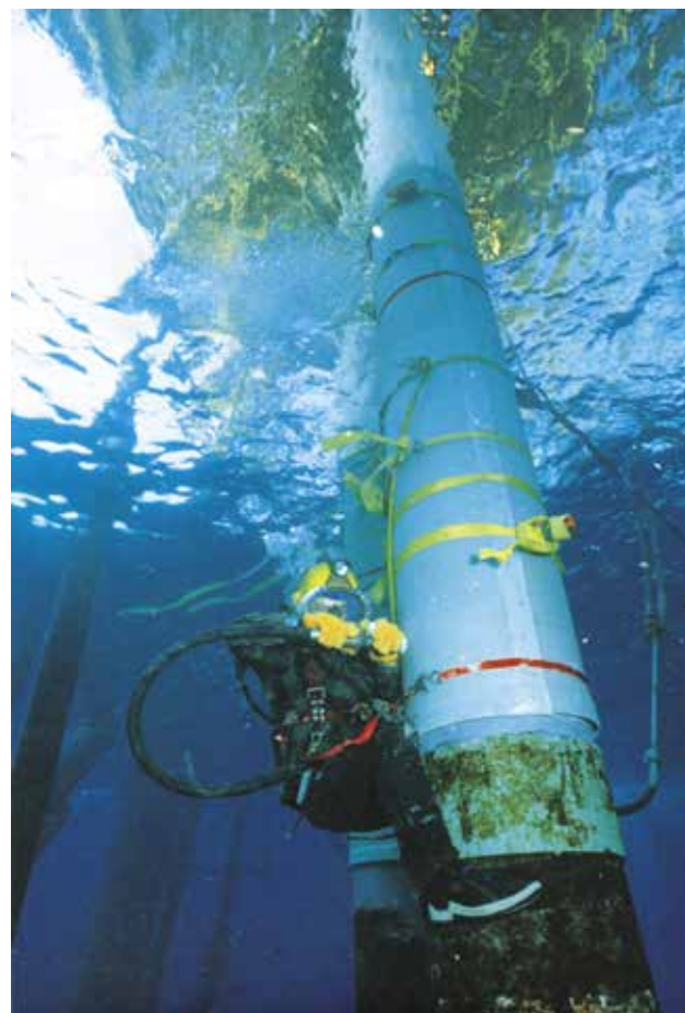
BASF's underwater grouting technologies help to protect bridges against seawater corrosion.
