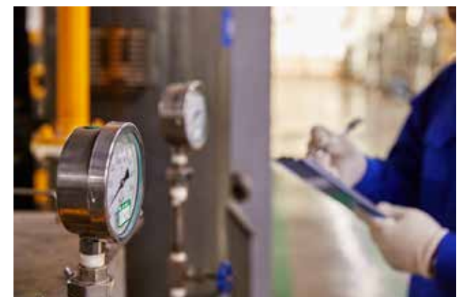
Inspection of pressure in the production facility
