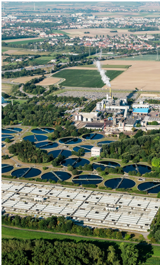
The BASF wastewater treatment plant at the Ludwigshafen site in Germany is one of the largest in Europe. Around 86 million cubic meters of production wastewater are treated here every year, plus around 18 million cubic meters of wastewater from surrounding communities. In recent years, we have continuously increased the energy efficiency and effectiveness of the plant.
