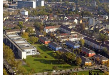
View from above: the LUWOGÉ Brunck residential quarter in Ludwigshafen.
