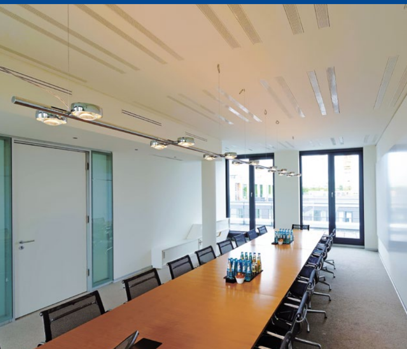
Full Integrated, thermally active ceiling Ceiltec® with strip absorbers made of Basotect®, Innogration GmbH, D
