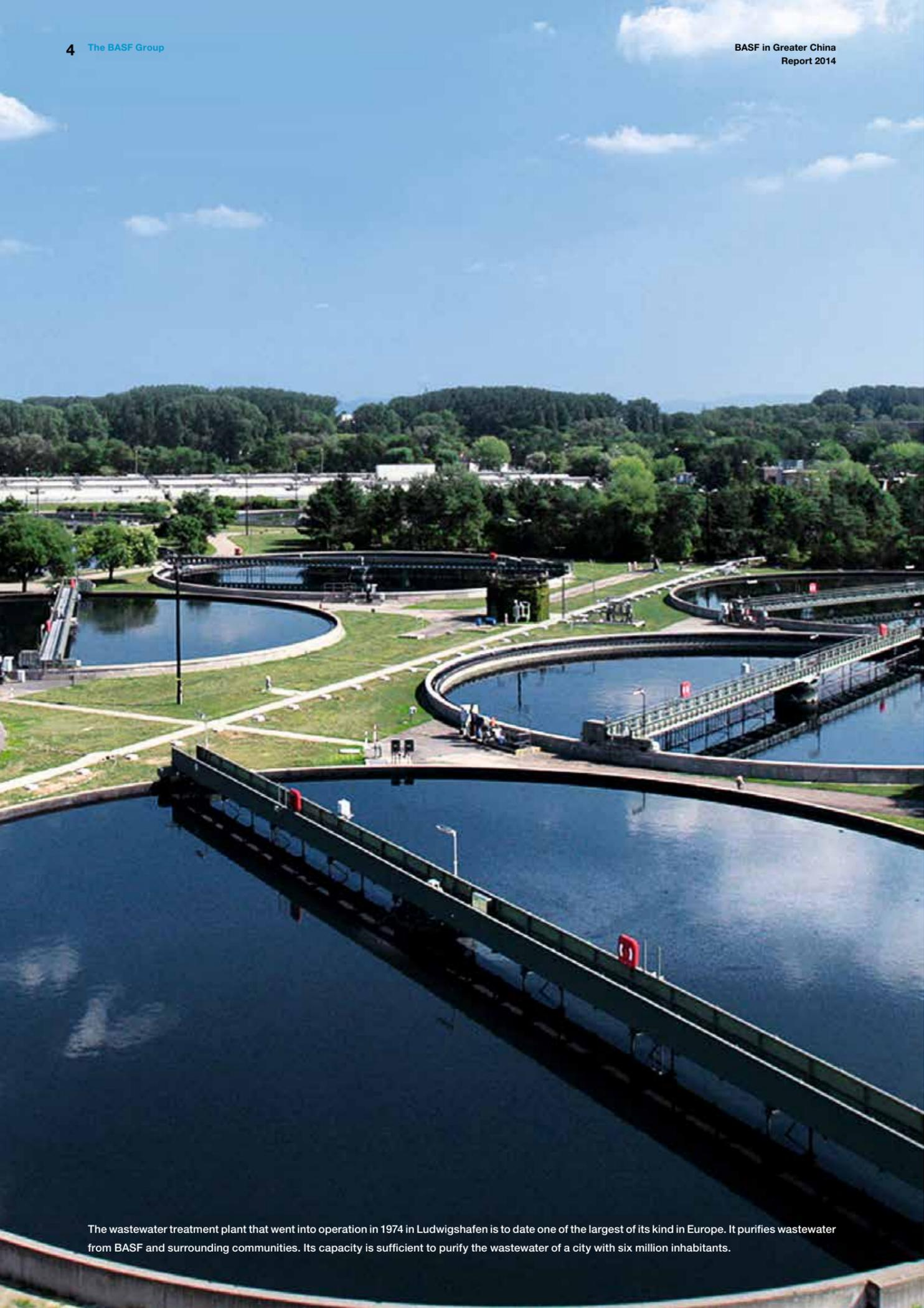
The wastewater treatment plant that went into operation in 1974 in Ludwigshafen is to date one of the largest of its kind in Europe. It purifies wastewater from BASF and surrounding communities. Its capacity is sufficient to purify the wastewater of a city with six million inhabitants.
