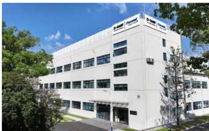
The Chemetall Innovation and Technology Center is BASF's first regional center for applied surface treatment technology in Shanghai, China.
