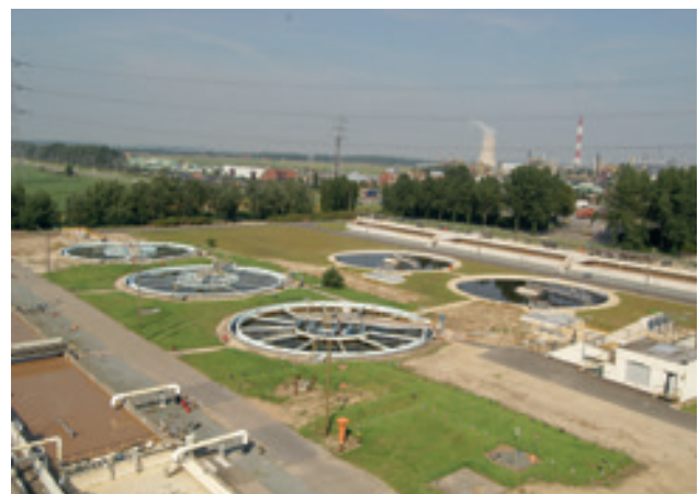
Our water treatment plant has the capacity to handle the waste water volumes of a city like Antwerp.
