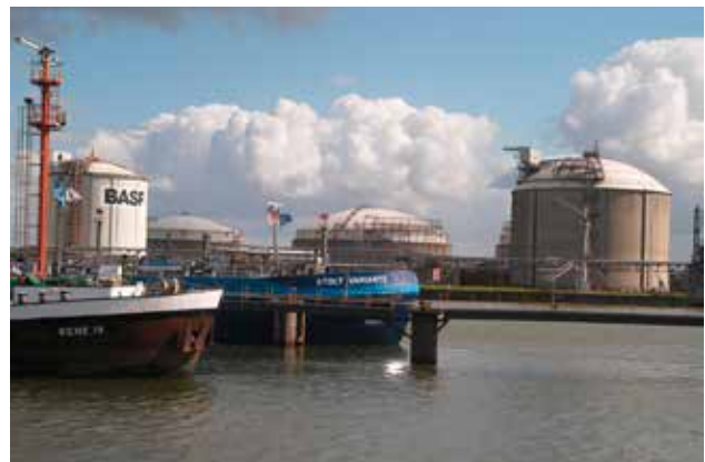
BASF Antwerp takes advantage of an ideal location close to many waterways, railroads and highways.
